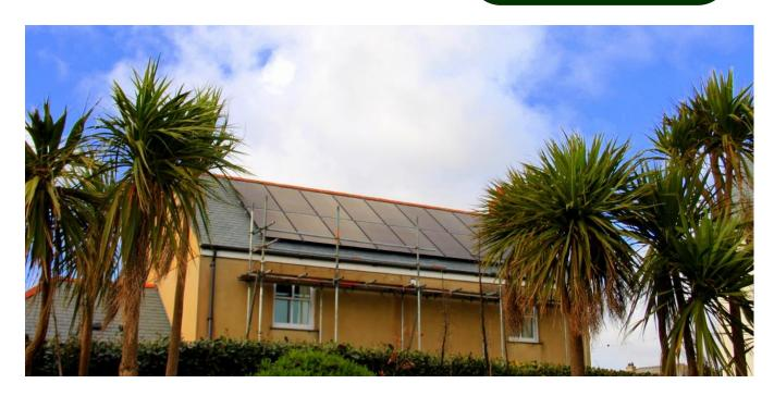
A Slate Mounted Solar PV system installed near Lands End, Cornwall using Black SolarWorld Modules.
